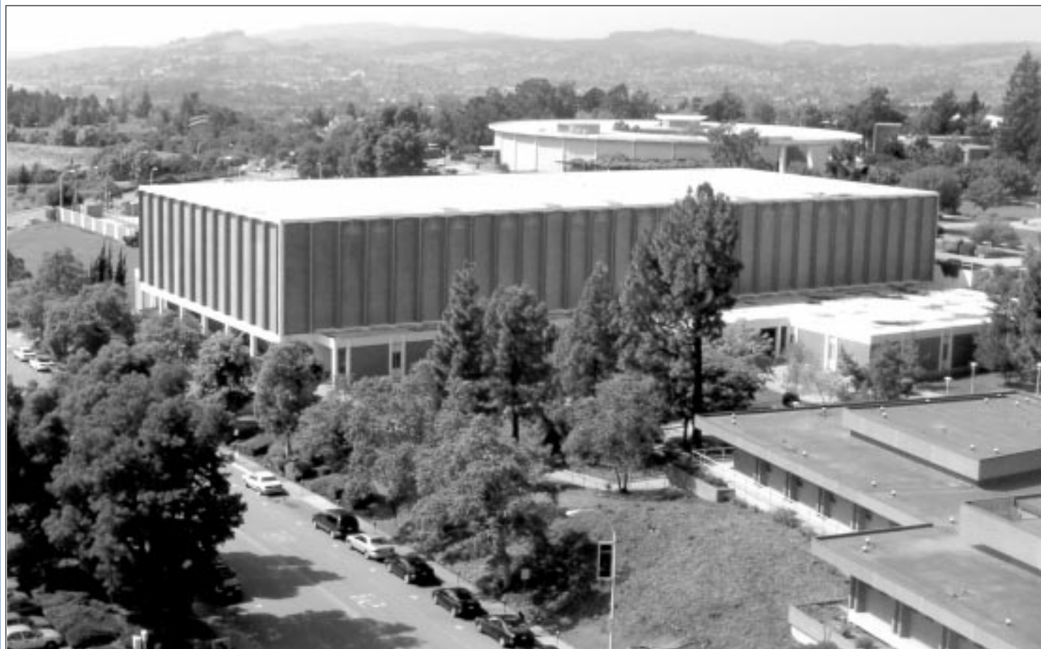
Rooftop Energy: The roofs of the Cal State Hayward gym and Music and Building (circular structure in background) as well as that of Meiklejohn Hall, soon will support solar power systems.
